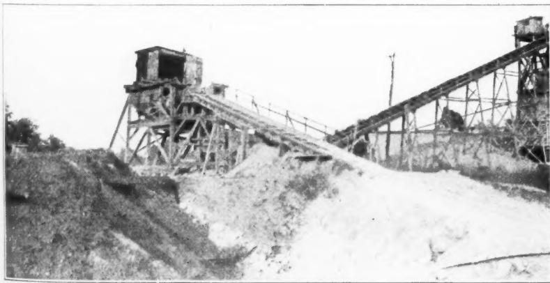
Incline At Top of Which Cars Are Dumped Into Hopper Which Feeds Material to Scalping Screen
